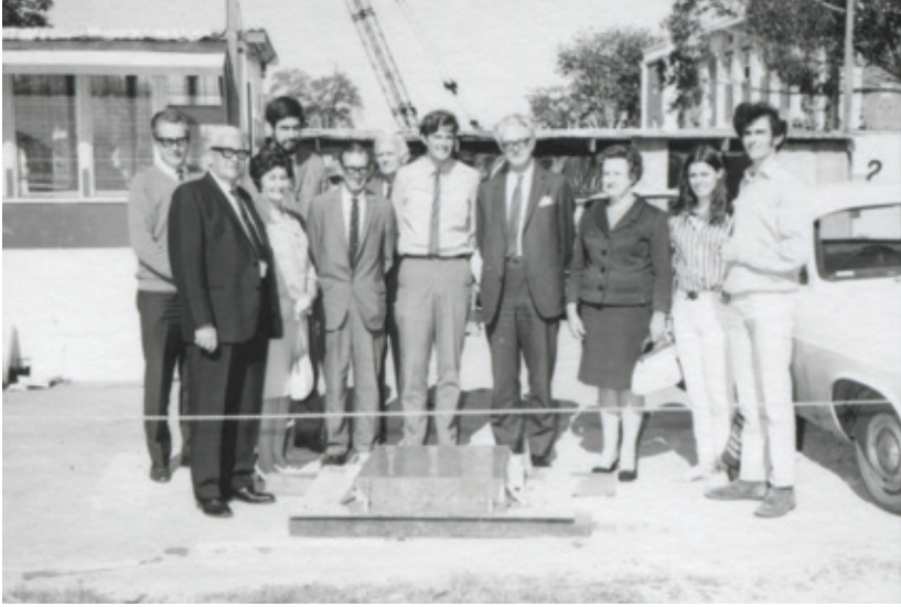
K.Beazley - Laying Foundation Stone New Guild Building 1970
