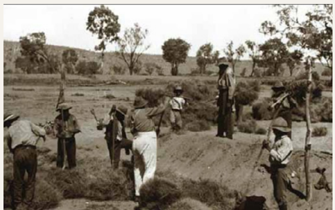
Left: Sources of Spinifex distribution in Australia [PhD Thesis [pag 34] Right: Workers laying spinifex during road construction in Central Australia 1912-1951. Photograph is part of the Australian Inland Mission Collection (nla.pic-an24666817). [Image courtesy of National Library of Australia].
