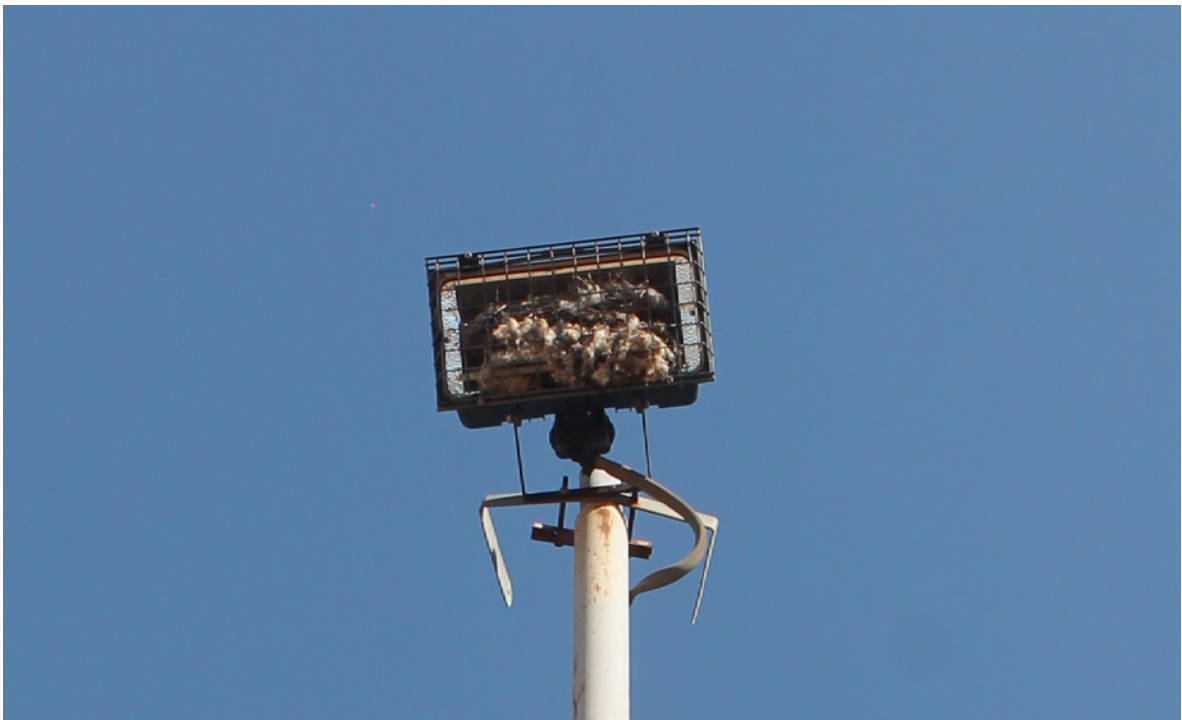
Figure 64: Existing floodlights are damaged and inoperable
