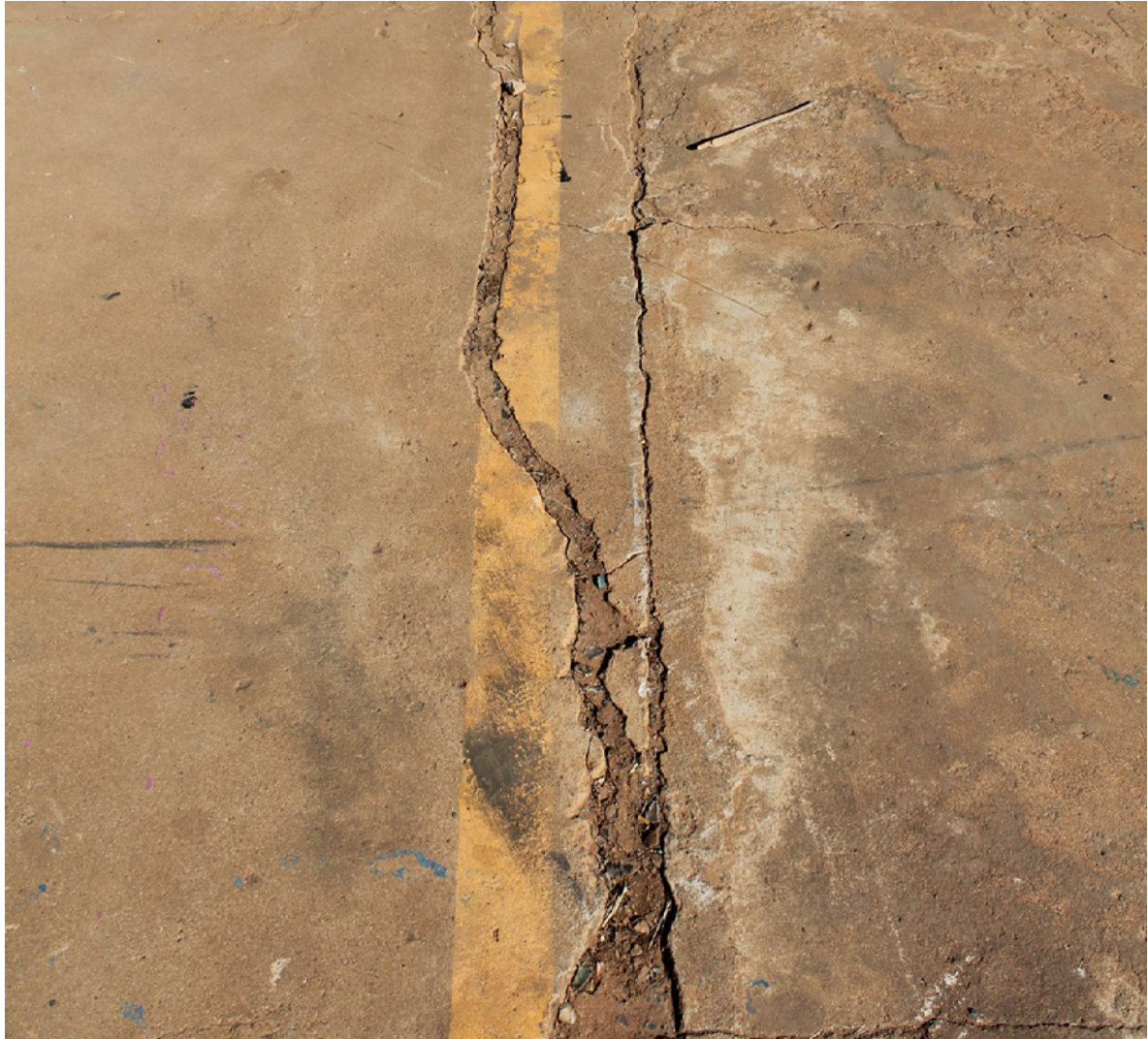
Figure 48: Cracks on court
