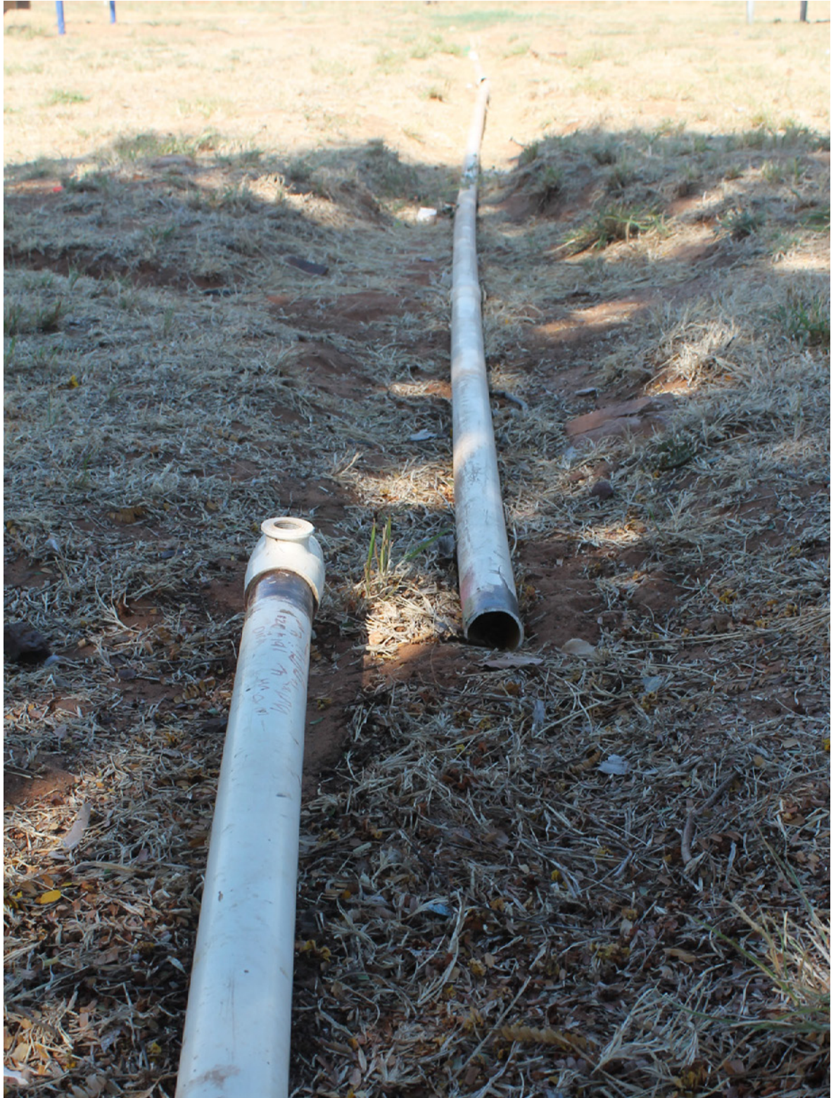
Figure 77: Abandoned and disconnected water pipes
