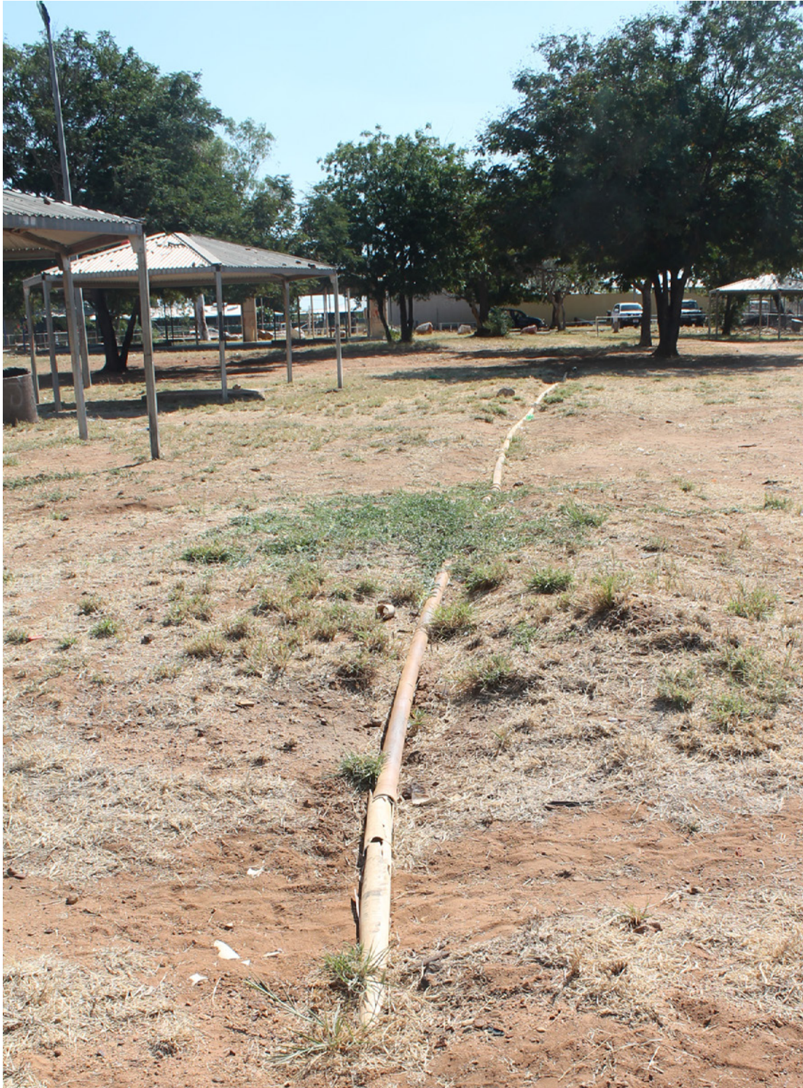
Figure 78: Exposed water pipes located next to courts
